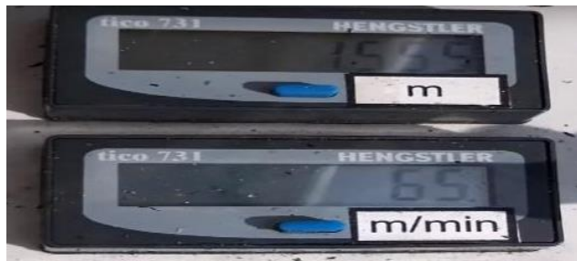
Fig. 4.32: Meter shows the distance and speed of the cable into the micro duct
