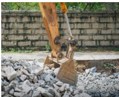
Fig. 4.3 Removing of Rocks and sharp stones during the trenching
