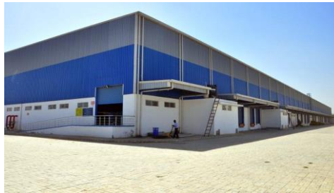
Fig. 1.18: Warehouse storage and ventilation
