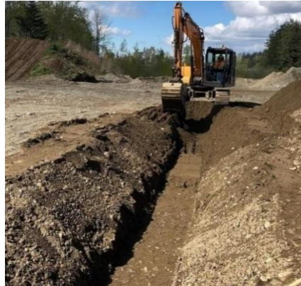
Fig. 4.10: Slope in the trench
