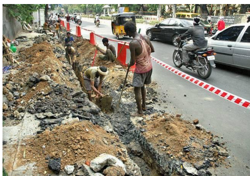
Fig. 4.5 Photo shooting Manual digging in an urban area
