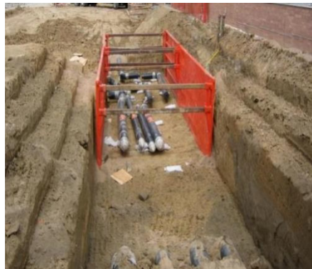
Fig. 4.11: Bench in the trench
