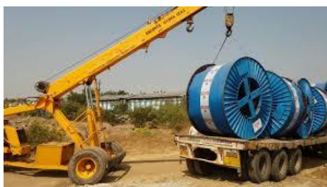
Fig.2.2: Crane carrying Cable Drum
