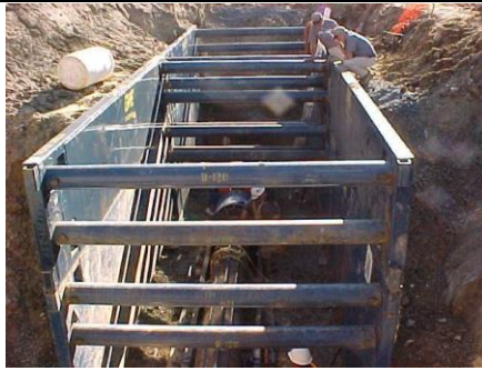
Fig. 4.9: Shielding of trench
