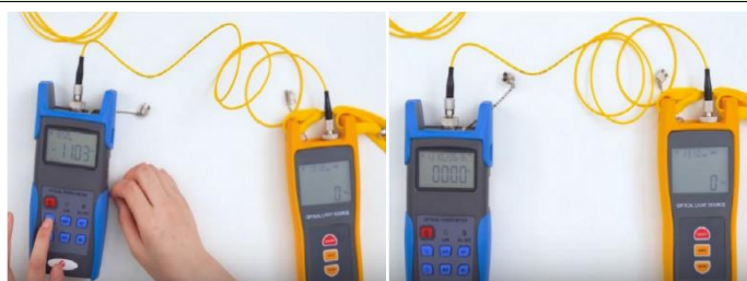
Fig. 3.7 Setting up the optical power meter and light source
