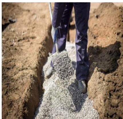
Fig. 4.33: Refilling the trench
