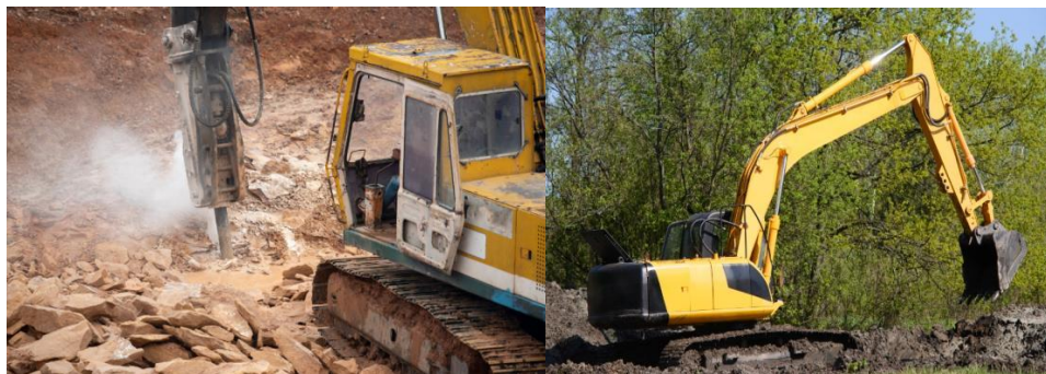
Fig. 1.14 (a) Excavation in rock (b) Excavation in forest
