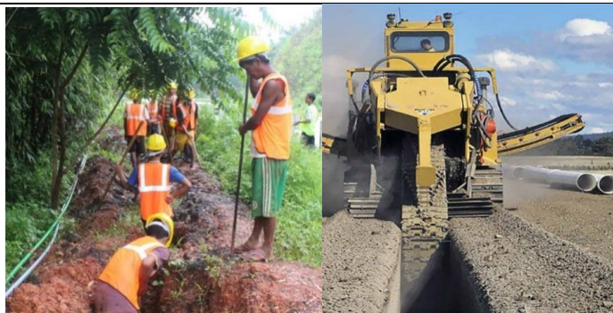
Fig. 4.2 (a) Trenching using hand tools (b) Trenching using machinery
