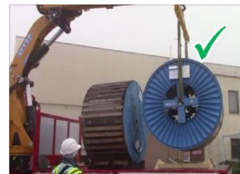
Fig. 2.7: (c) Way to lift and place the cable drum
