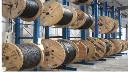
Fig. 2.18: Cable drum in the warehouse
