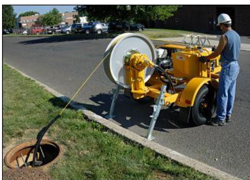
Fig. 4.20: Pulling machine pulling the optical fibre cable
