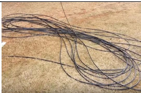
Fig. 4.18: Right way of placing the cable
