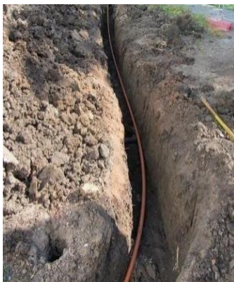
Fig. 4.13: Placing the cable in the trench
