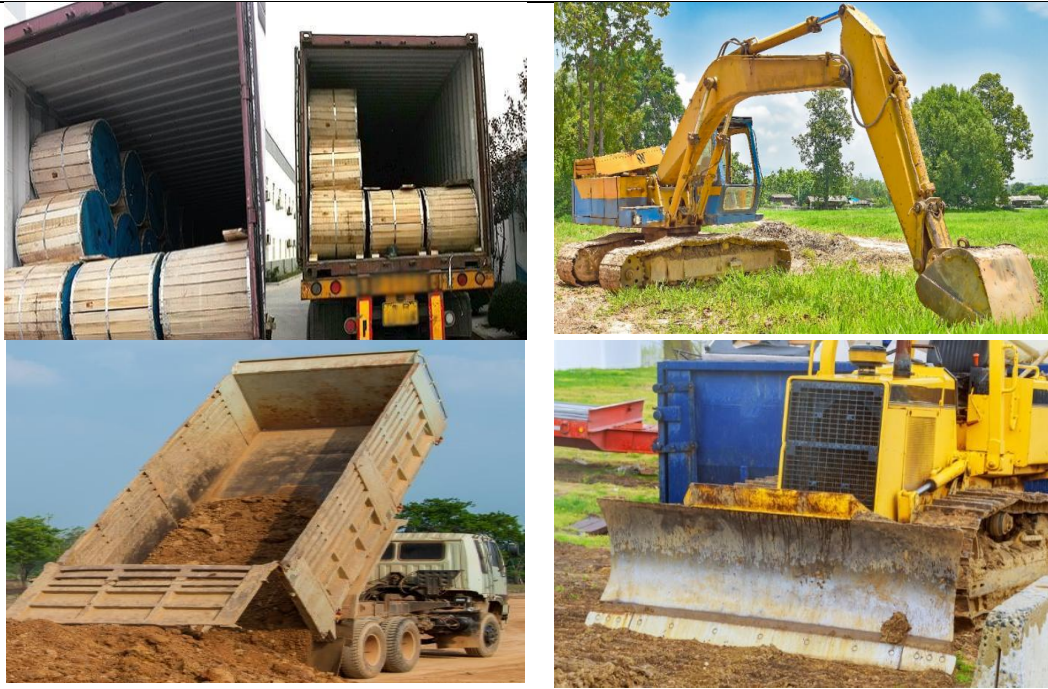
Fig.1.17: Transport vehicles involved in the OFC installation
