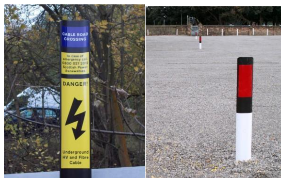
Fig. 4.34: Route marker and warning tape on the ground surface
