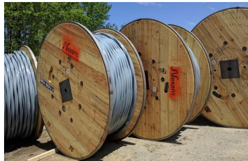
Fig. 2.19: Correctly organised cable drums
