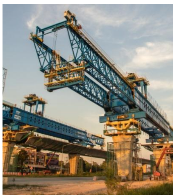
Fig.1.15: Mega structure highway project
