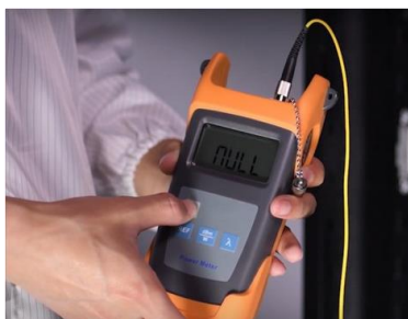
Fig. 3.2 Connecting optical fibre cable to its port
